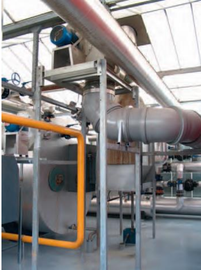
Figure 1. CO 2 burner enriches the glasshouse environment, so helping provide an optimum growing environment. (Biocyclopedia), https://biocyclopedia.com/index/principles_of_horticulture/photosynthesis.php .
